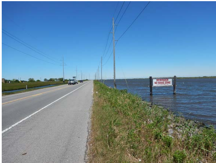
“No Wake Zones” are important, as boats traveling too fast will etch away The narrow soil areas that protect LA 1.
