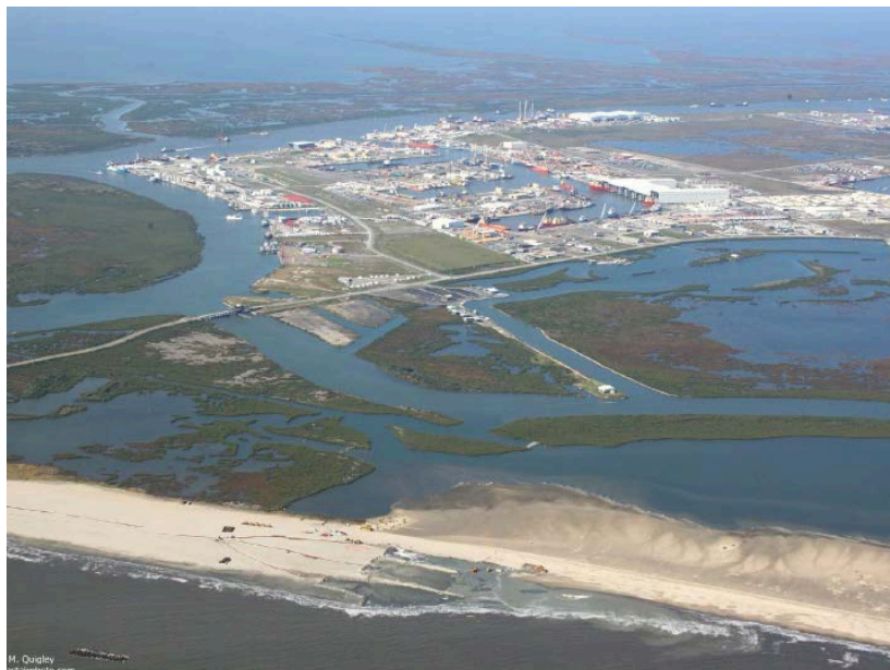
Port Fourchon in the rear, and note the pipeline in the center of the beach to the left that forks to three pipes that deliver the sand. Note how wide the nourished beach is to the left as opposed to the soon-to-be nourished beach to the right where sand has progressively moved north into the estuary.
