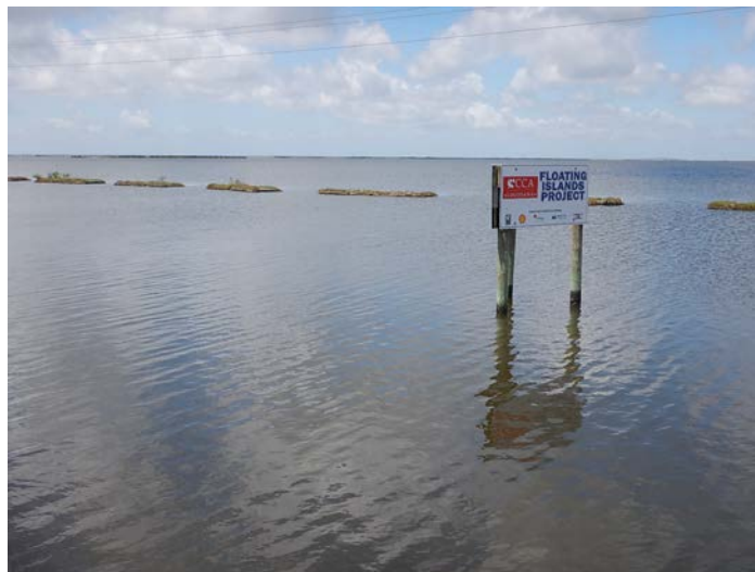
Floating Island Project along LA 1 between Fourchon and Grand Isle.
