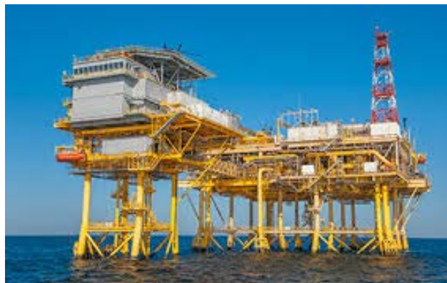
The LOOP offshore facility that oversees the offloading. Loopllc.com.
