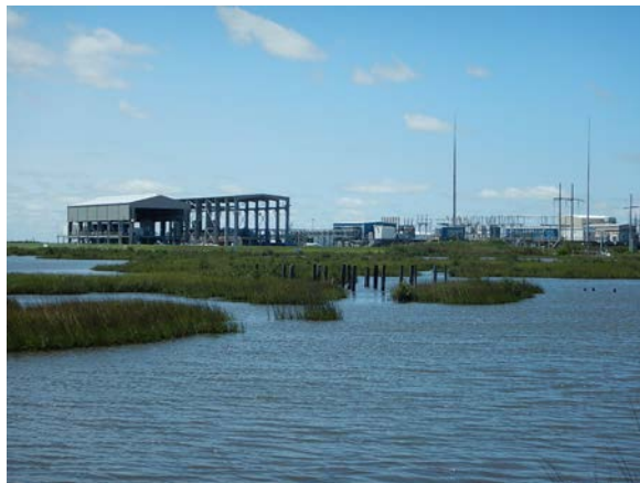
LOOP booster station.
